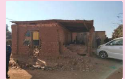
Police station before renovation
