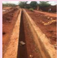
Drainage ditch in KAMATETE
