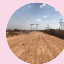
KASAPA road repaired by CDM
