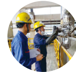
Site of skill standard practical operation
