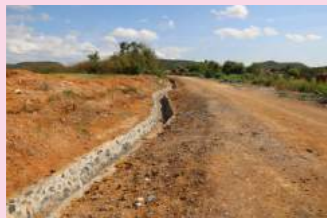
Drainage canal beside road after construction
