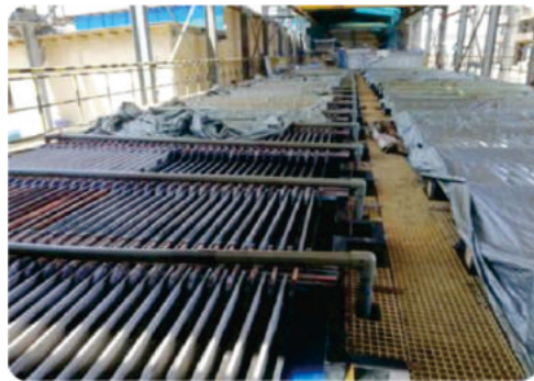
Completed installation of acid gas recovery pipeline
