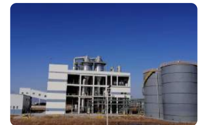
Desalination treatment plant of high salinity wastewater in Huajin
