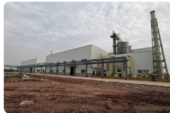
Homogenization and dewatering treatment project of solid waste center of Quzhou Huayou
